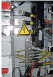
In order to reduce system-related network repercussions and increase machine availability, the drive system is fed by an IT system which is determined by a transformer without a neutral point and is therefore unearthed. For this reason, the
